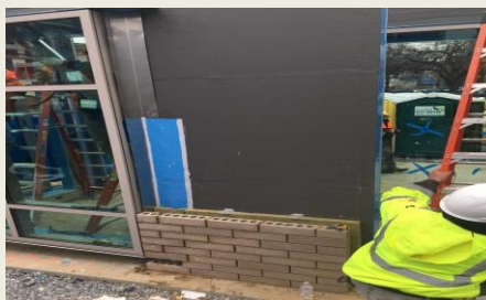
Exterior Mock Up
