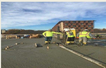
Installation of 4th floor deck
