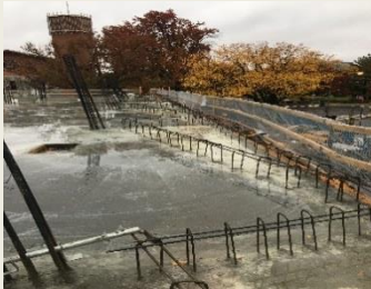
Installation of 2 nd floor deck
