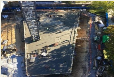
Install of 1 st Floor Deck
