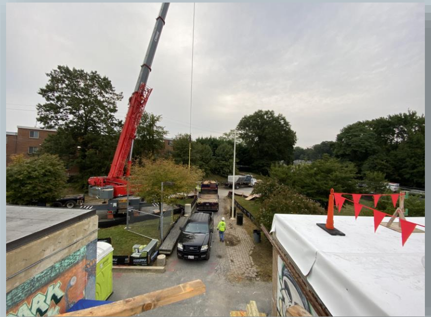
New Roof is being installed
