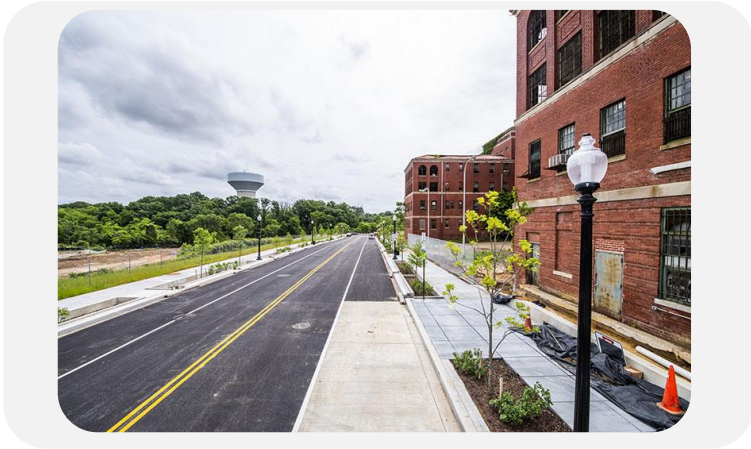
St. Elizabeth's East Campus 2023 CMAA Project Achievement Award
